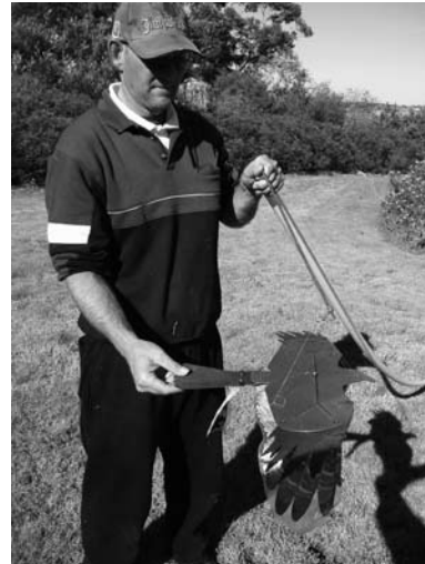
4) Tie the hawk to the bent arm of the reinforcing by tying line to three holes in the hawk's head and back of each wing.
