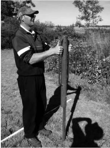
1) Ram a steel post into the ground.
